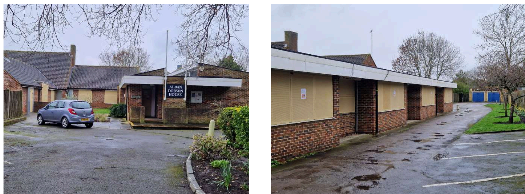
Existing site photographs
